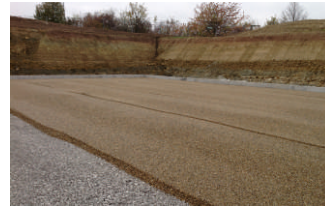
Subbase and base course
